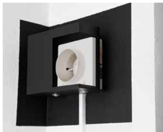
fig.6 Unwanted darkroom odors are effectively removed with a regular extractor fan and a custom-made, light-trapping air-path, which is illustrated here by a cut-away.
